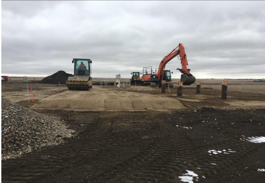
Compacting pad valve#7 SSKP 298+877
